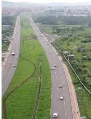
Greenery for highway junctions and crossroads
