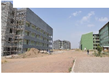
Campus Building Construction
